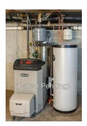
Built on the Weil-McLain® Ultra Oil (UO) Boiler with Taco® Delta-T Circulation
