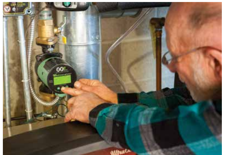
SYSTEM SETUP: Mercier sets system delta T performance.
