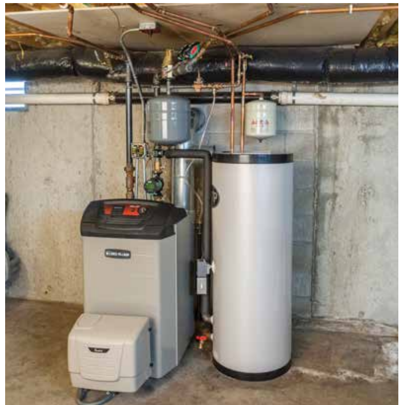
THE FINAL PRODUCT: Appliance installation completed.
